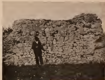
4 A PIECE OF THE MURO PERTUSO BETWEEN TWO BUTTRESSES View from the south
